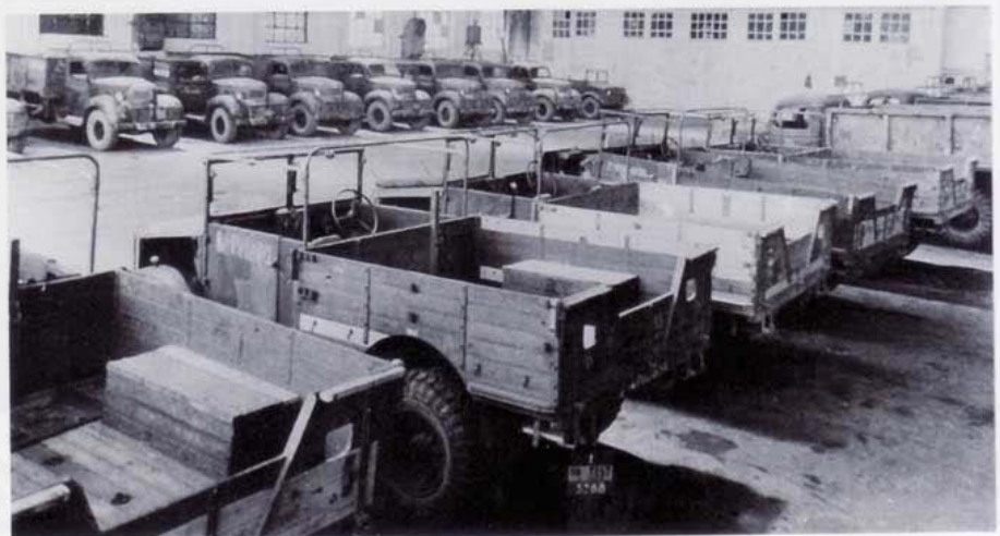
This vehicle was issued for driver training early in the war. Note the radiator cover on the front bumper. As can be observed, very little weather protection was given to the cab and even less was provided in the body area. An Austin 8hp two-seat car can be seen on the right.
