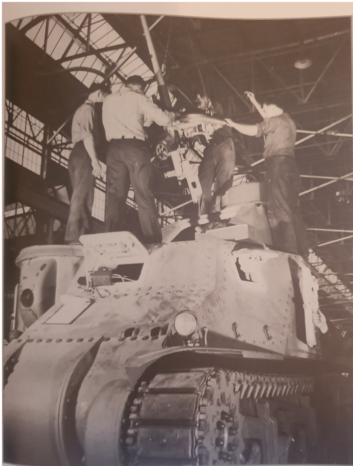
Above: Several workers are guiding a 37mm gun mount into its position on the front of the turret of a Chrysler Medium Tank M3. The gun is viewed from the left side, also showing the recoil guard and the elevation hand wheel. Note the white paint overspray on the exterior of the hull around the driver's vision port and the pistol port. Library of Congress
